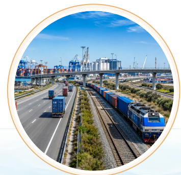
External connectivity infrastructure
